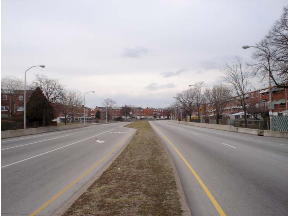
Figure 21: Housing Separated by Lindbergh Boulevard
