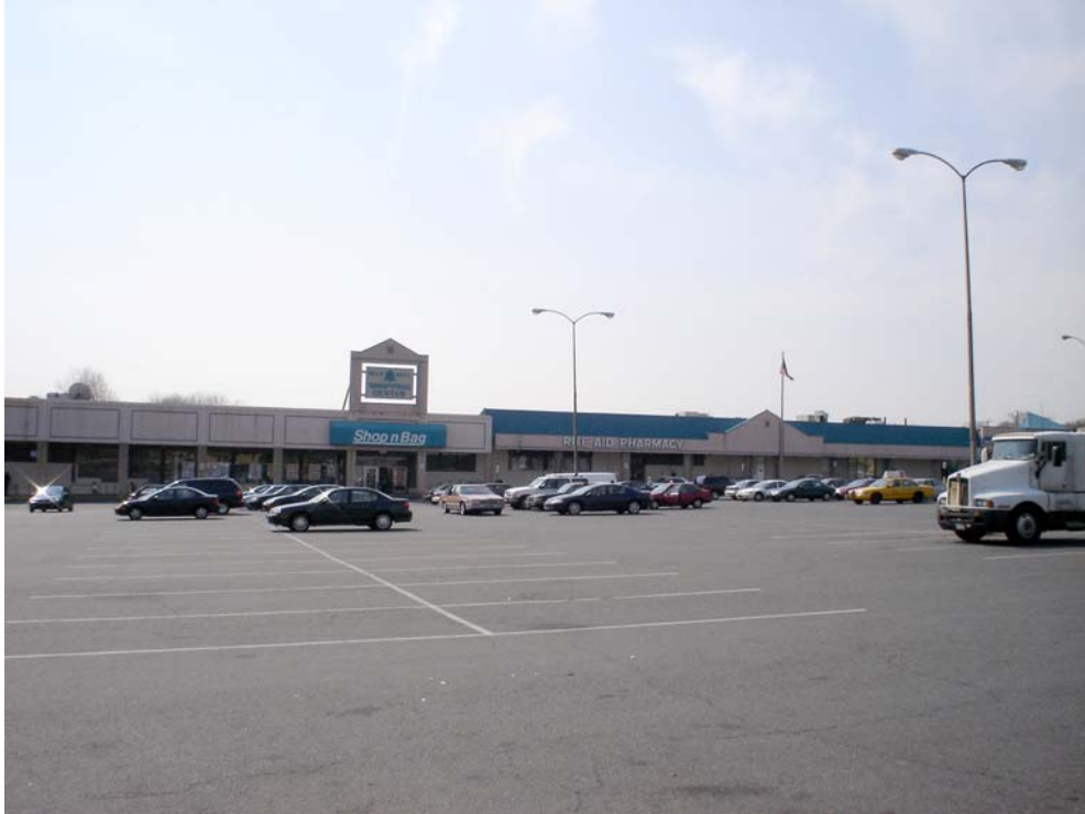
Figure 23: Suburban-Style Neighborhood Shopping Center on 70 th Street
